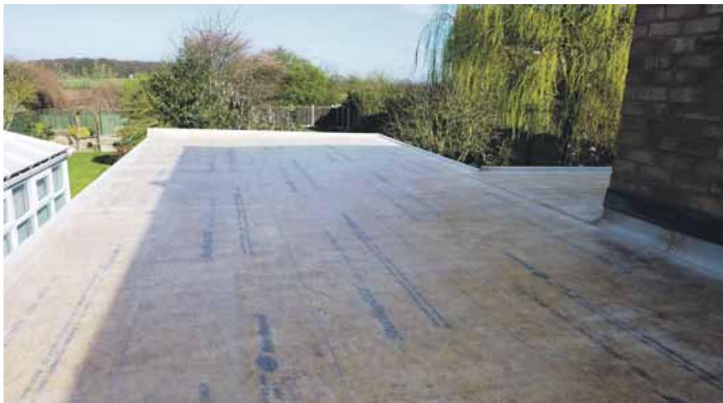
Fully laminated roof - laminate is transparent. Note writing on deck
