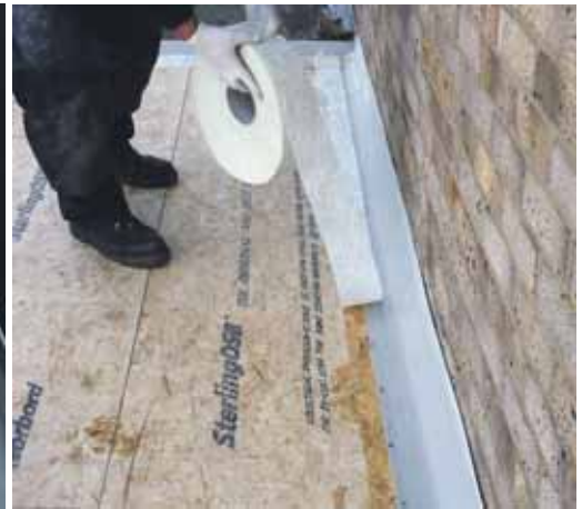
Bandage laid into resin
