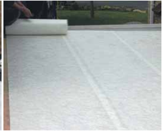
Continue overlapping each strip by 50mm
