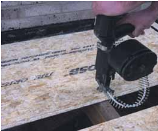
Decking fixed to support joists
