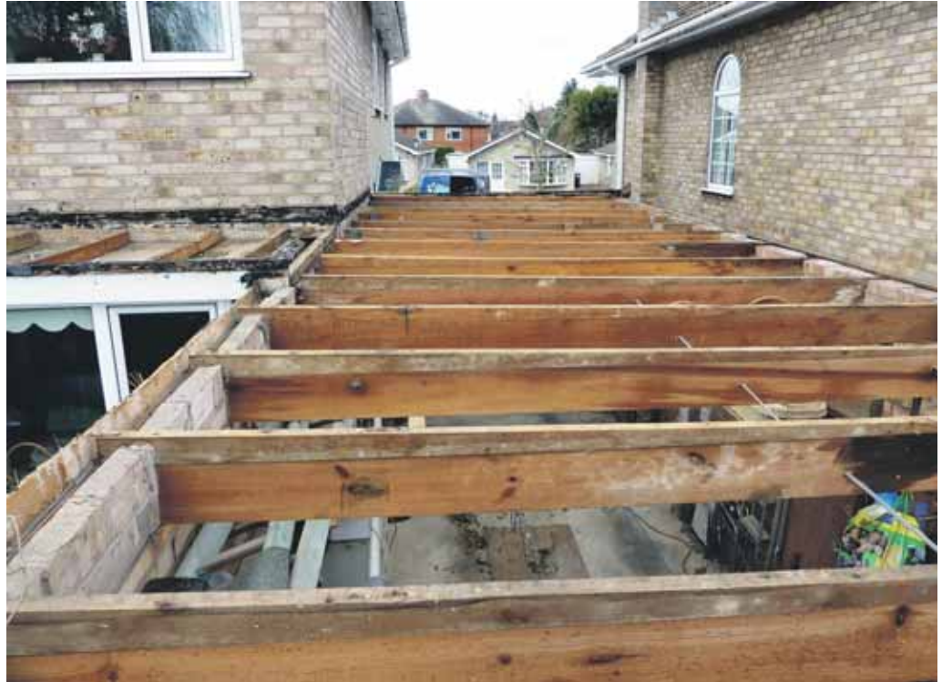
Roof stripped showing furrings on top of joists
