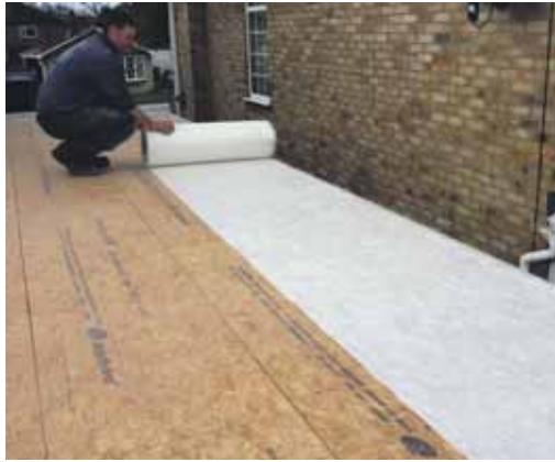
Lay out first strip of mat along lowest point
