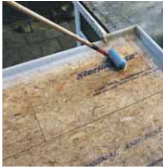
Base resin onto deck
