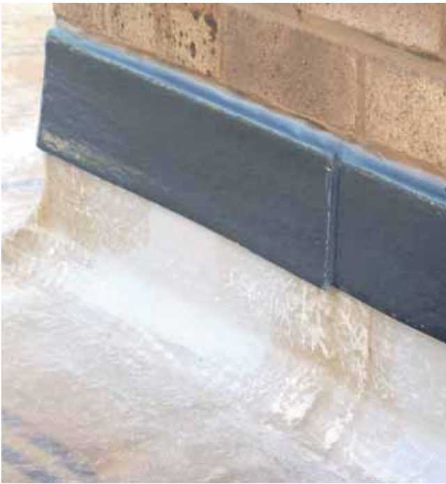
Flashing in place. Laminate sanded ready for top coating
