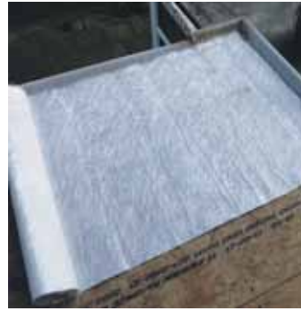
Mat laid into resin
