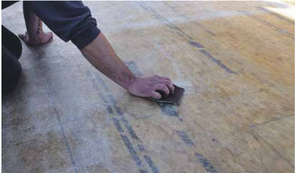
Lightly sanding cured laminate
