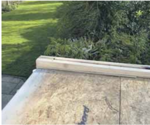
Reverse furring to level front and rear elevations
