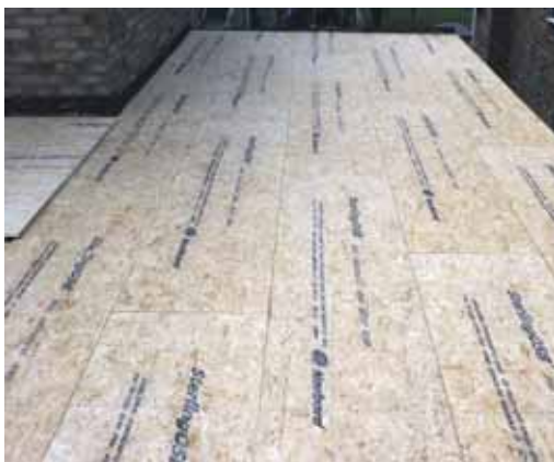
Decking laid - writing side up
